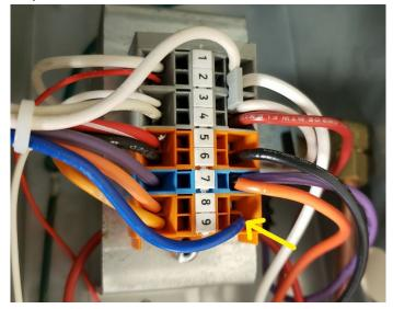
2. Connect supplied blue wire to the Ignitor 500VA terminal on oil primary control.
